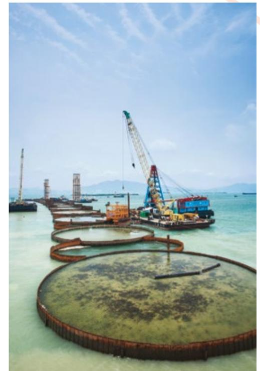
The composite section of the seawall was constructed using a series of 32m diameter steel cofferdams
