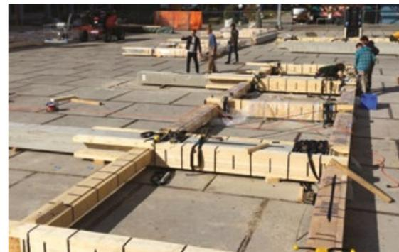
The frames were first constructed on the ground and then hoisted into place
