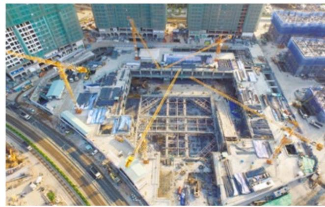
Site photo showing the central zone (bottom-up method area) and perimeter ring slab (top-down method area). The photo also highlights the space constraints of the site.
