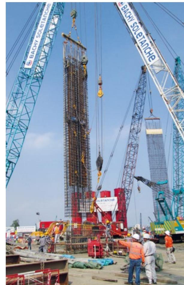
■ Installation of the reinforcement cage of a barrette pile
