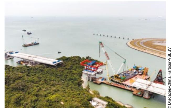
A tailor-made straddle carrier was used for bridge deck erection across the Sha Lo Wan Headland
