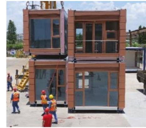
■ The module under fabrication in the factory (left) and a trial assembly carried out before shipping (right)
