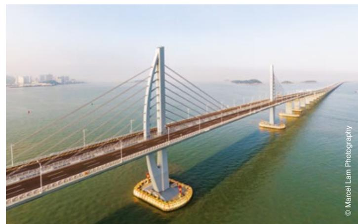
Jiuzhou Channel Bridge with sail-type towers. The form was proposed by Arup in the preliminary design.
